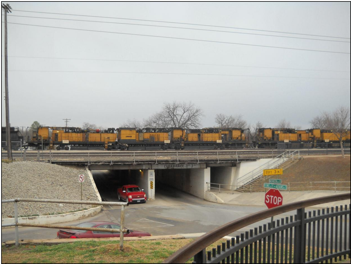
BNSF Track Maintenance Train used to upgrade line between Coleman and San Angelo
