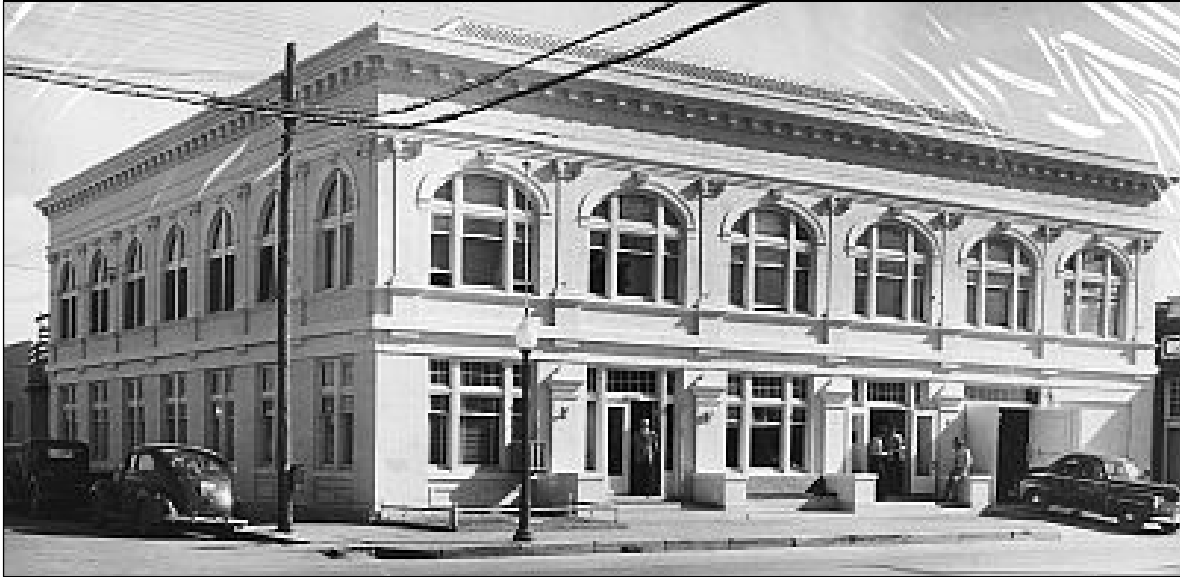
Brownwood City Hall and Fire Station
