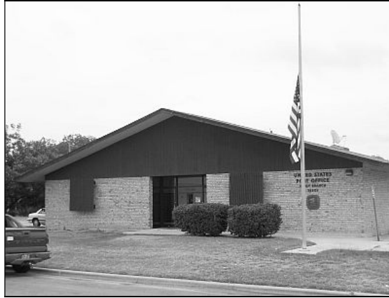
Early Post Office Sub-Station
