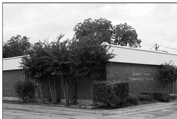
Adams Street Community Center
