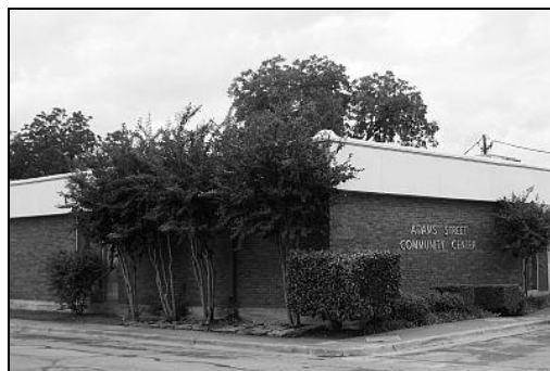
Adams Street Community Center
