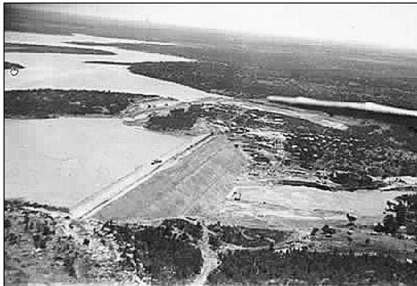
Lake Brownwood Dam in 1932
