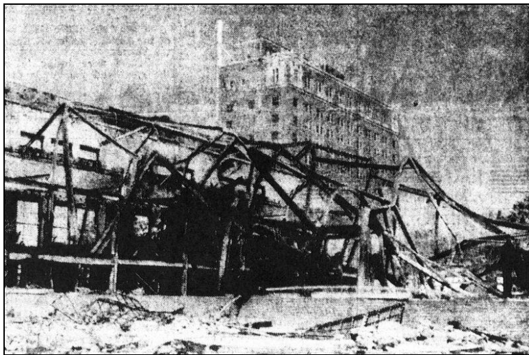
Twisted Steel Beams at Brownwood Memorial Hall
