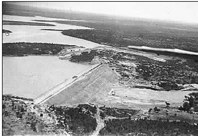
Lake Brownwood Dam in 1932
