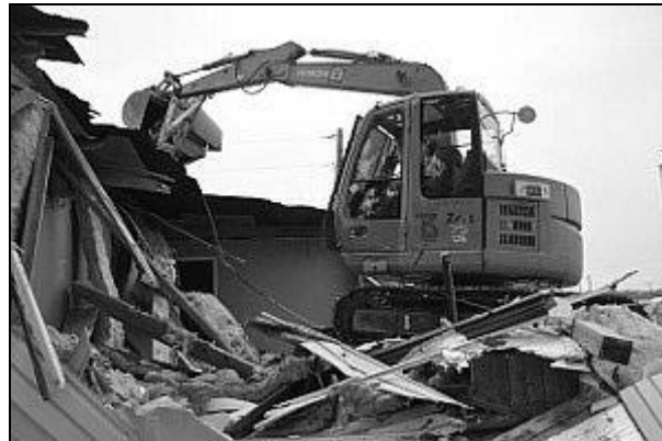
Red Cross Building Demolished
