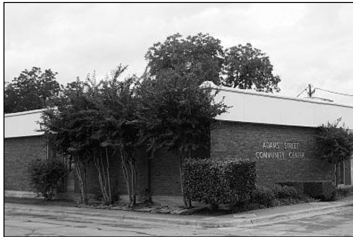
Adams Street Community Center
