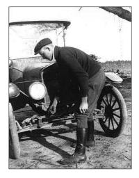
**First:** Make sure the gear shifting lever is in neutral position. **Second:** The clutch pedal is unlatched and the clutch engaged. The brake pedal is pushed forward as far as possible setting brakes on the rear wheel.
